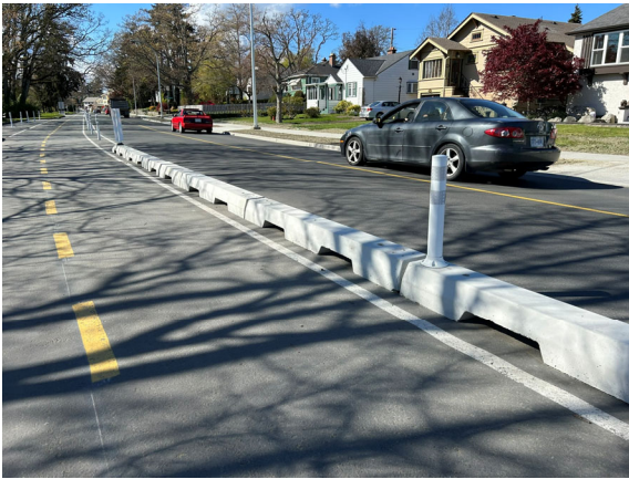
Examples of quick builds using concrete curbs (left) and plastic delineators (right)
