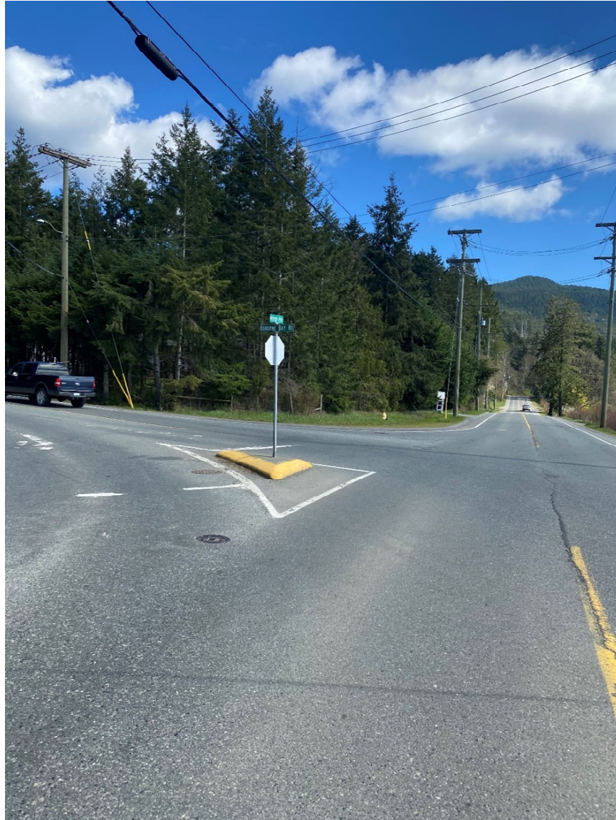
Example of a channelized right turn at the intersection of Osborne Bay Road and Herd Rd.
