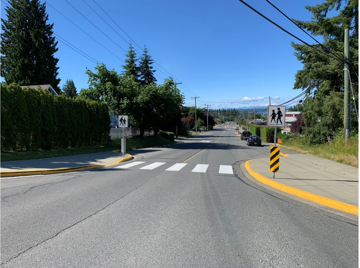
A crosswalk with curb extensions on York Avenue
